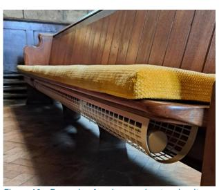
Figure 10 – Example of under-pew heaters in-situ at one of our churches.
