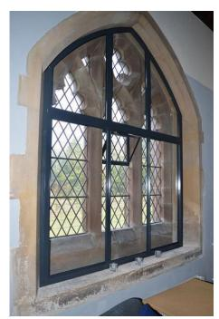
Figure 6 – Example of secondary glazing in a church.
