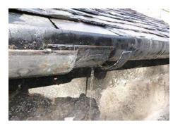
Figure 3 – Example of a leaking gutter
