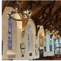
Figure 12 – Example of 'halo' infrared fittings.
